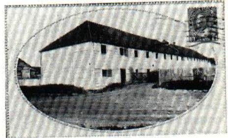
Part of Fort Edmonton before it was demolished.
