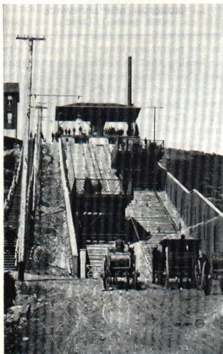
The Inclined Railway, which was used to transport vehicles from the bottom of McDougall Hill—Undoubtedly, the mail coach used this convenience.
