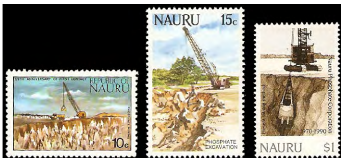
Excavation of Phosphate.
