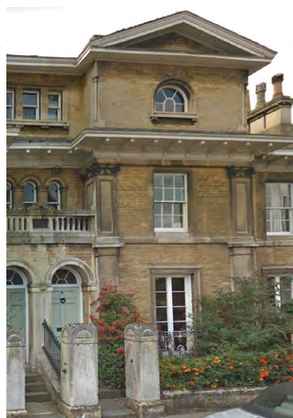
Figure 2. Rock Terrace, Stamford.
