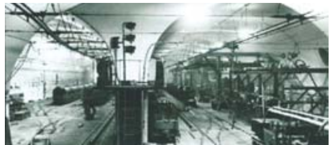
At the station approaches, the main tunnels divided into two 2.13 meter tunnels.
