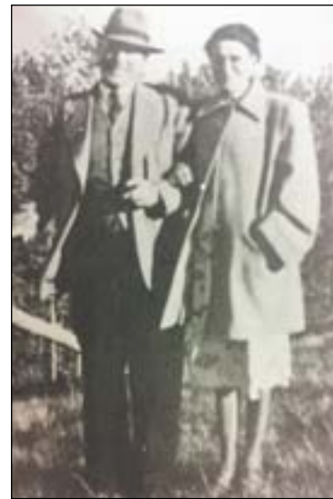
Figure 11 - East Coulee - Raisbecks
