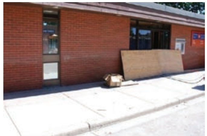
Figure 10 - close-up of flooded main post office.
