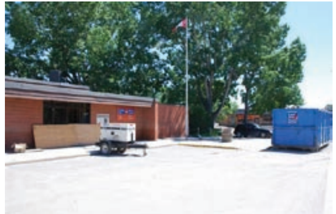
Figure 9 - flood damage, main post office.
