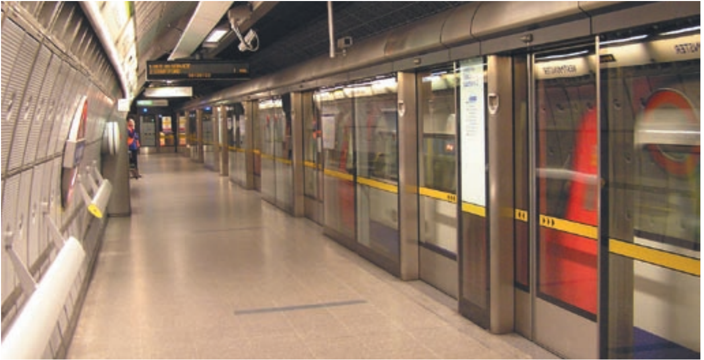
Fig. 13 Platform-edge doors at Westminster Station.
