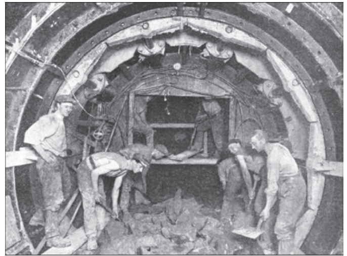
Fig. 9 Greathead shield.
