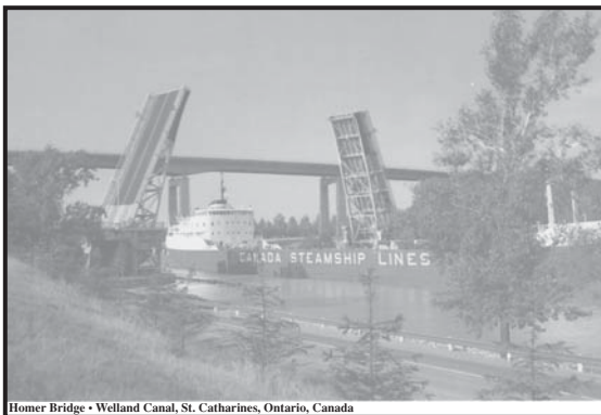
Homer Bridge • Welland Canal, St. Catharines, Ontario, Canada
