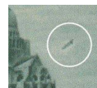
Spot at right of dome.
