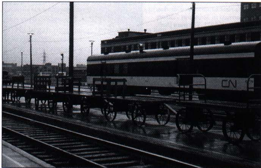
The end of the line: Mail car 7847 sits symbolically behind a row of empty mail wagons in Toronto's Union Station on the morning of 24 April 1971, following its arrival on Train 59 from Montreal. Thus ended a service that had operated continuously since 27 October 1856.
