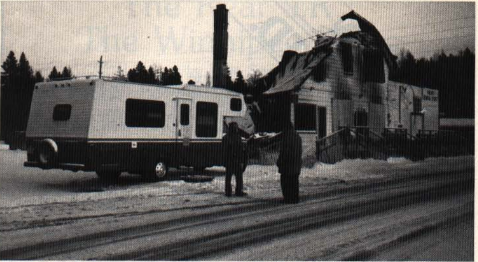
Mobile post office and burned out Tory Hill post office, Jan. 4, 1988.
