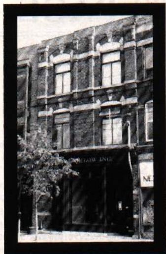
185 QUEEN STREET EAST
