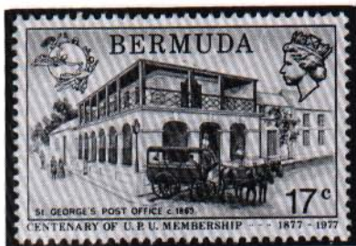
Fig. 9. St. George's Post Office, 1860 [Sc. 352, 1977]
